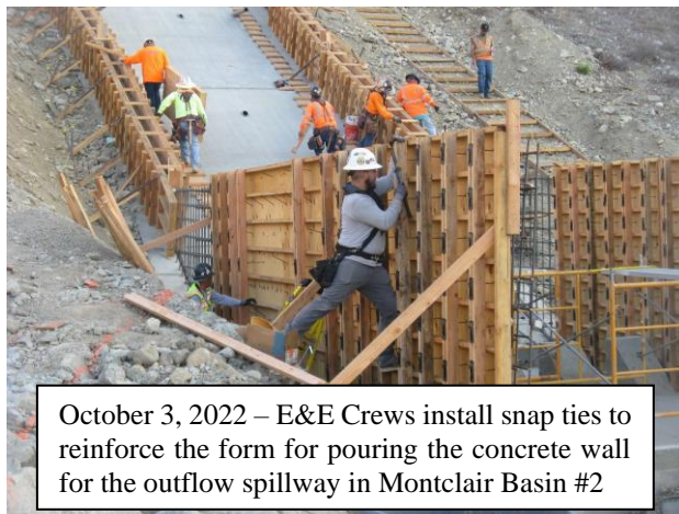
September 22, 2022 Rebar Placement and Building Concrete Forms for Walls of Spillway in Basin #2
