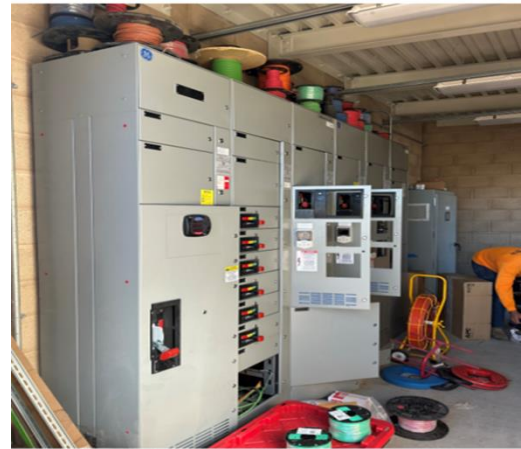
Installation of MCC Electrical Panel in EW-2
